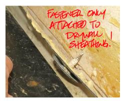
When scoping out the roofer and the CFMF and/or back of parapet sheathing contractor, make sure that either non-treated plywood or 20ga backing strip is properly being installed behind the sheathing.
